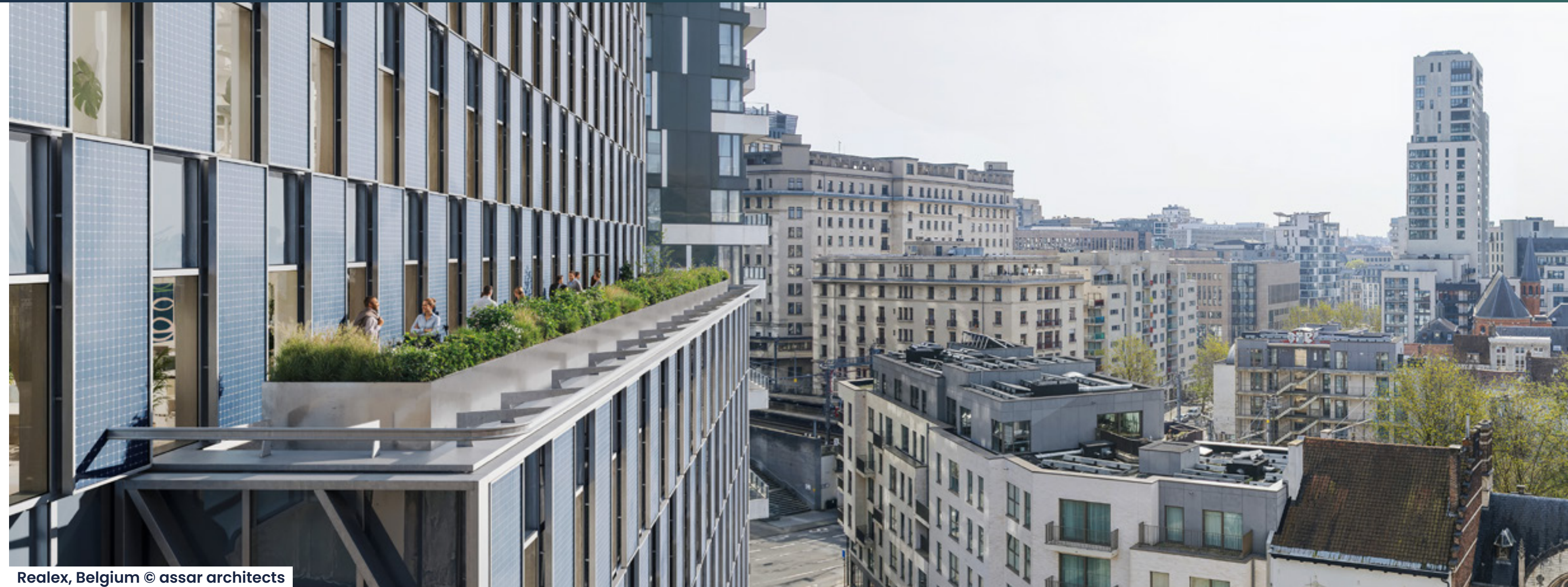
Realex, Belgium © assar architects
