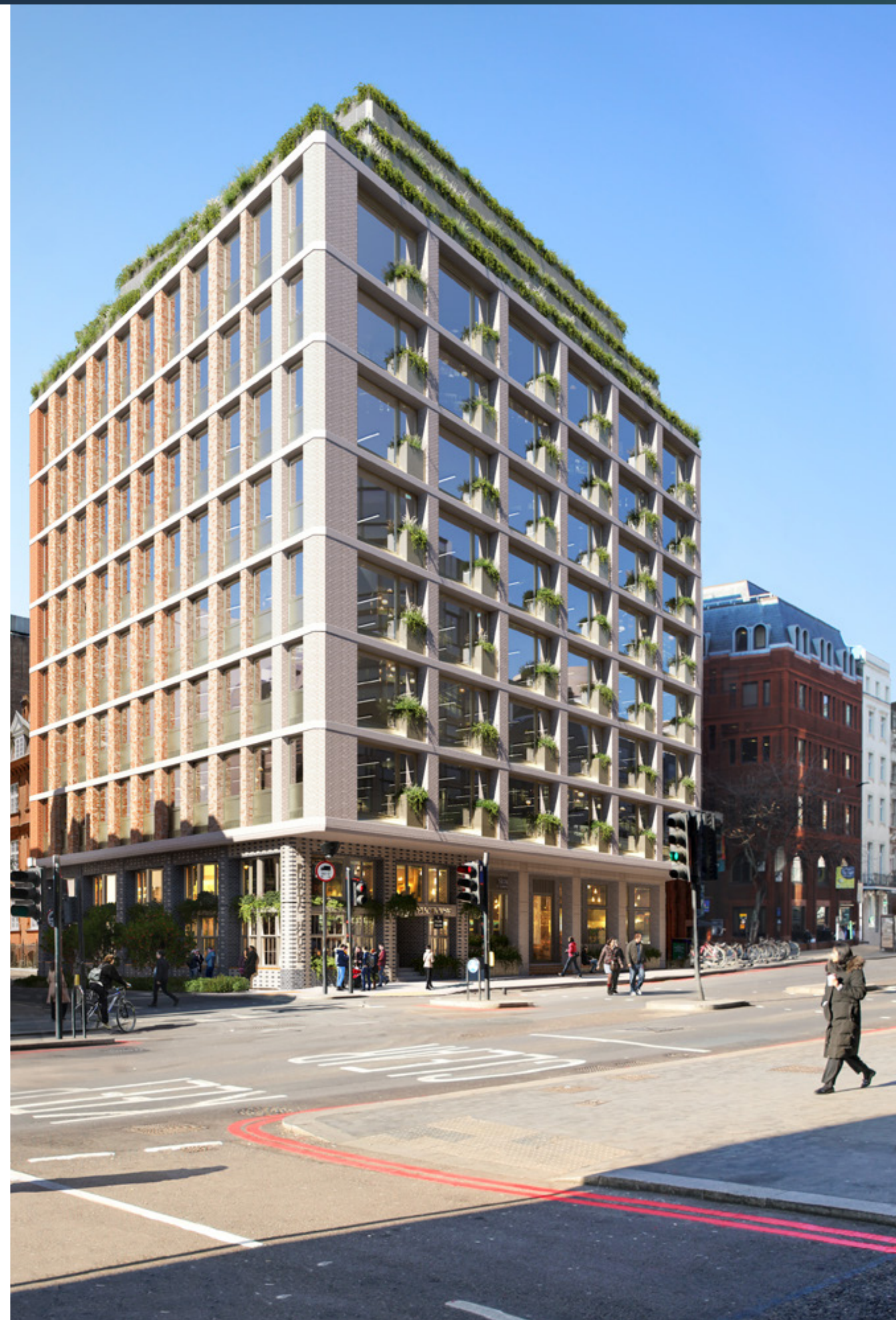
10 New Bridge Street, Royaume-Uni
