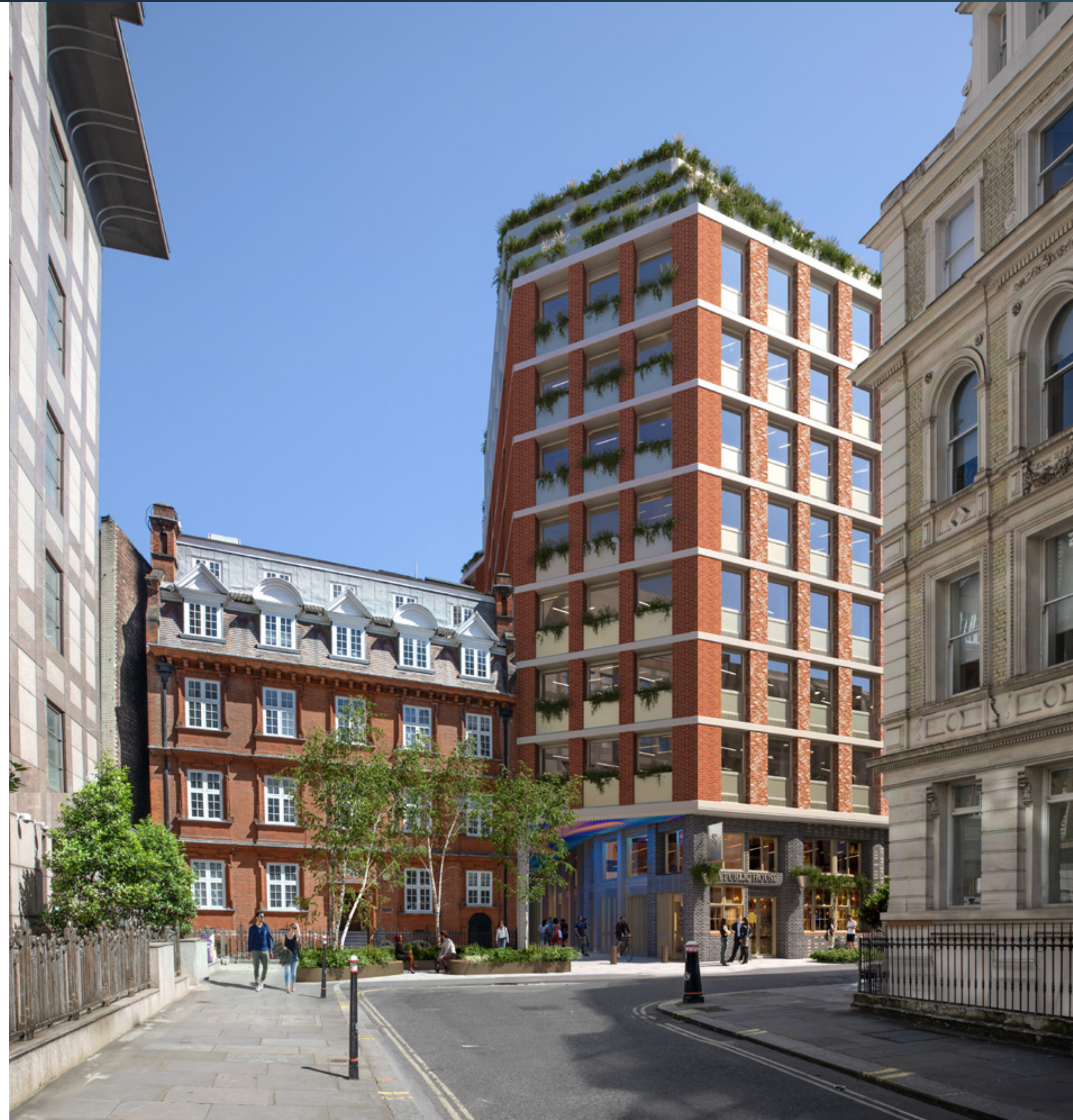
10 New Bridge Street, Royaume-Uni
