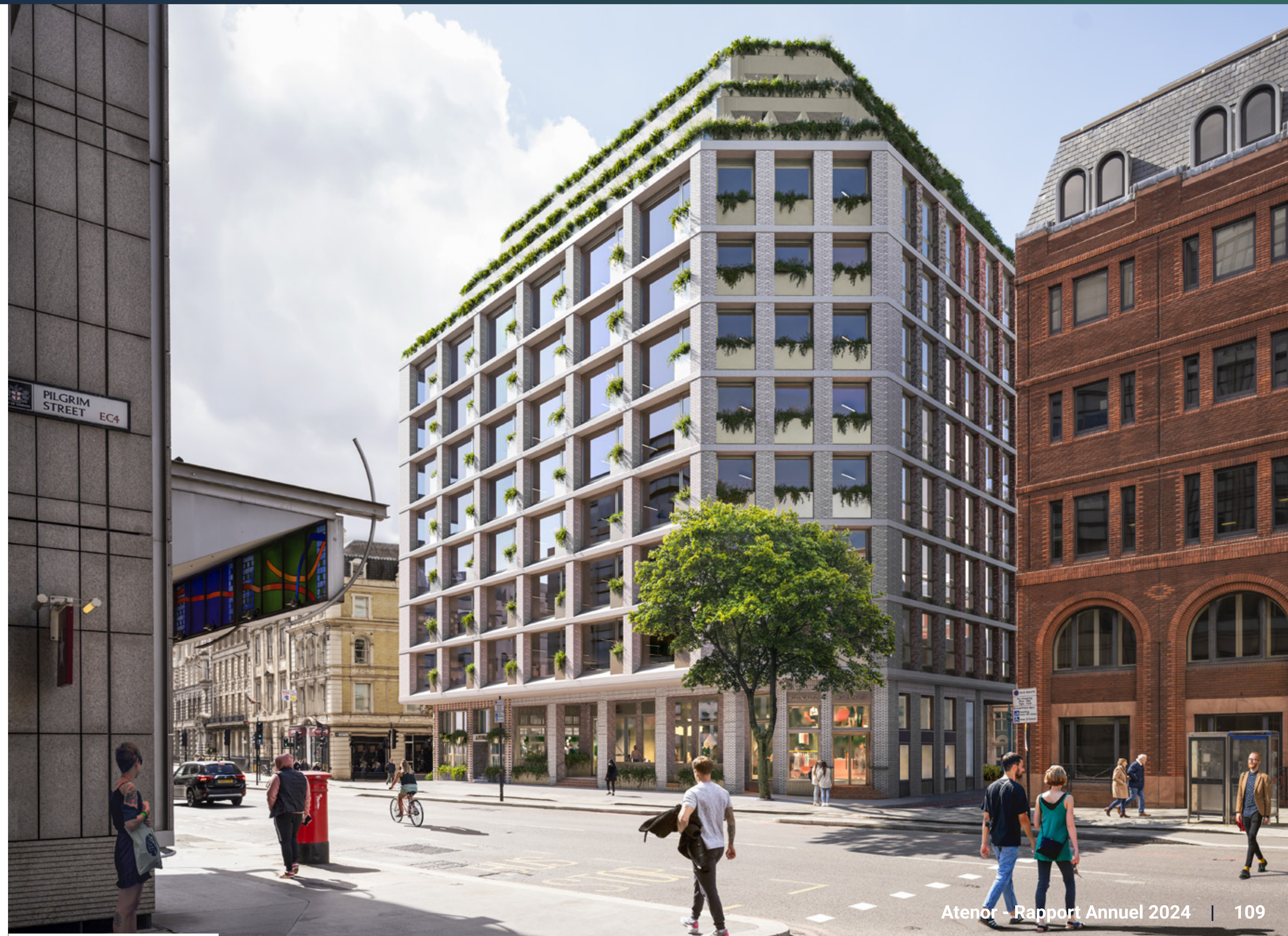
10 New Bridge Street, Royaume-Uni
