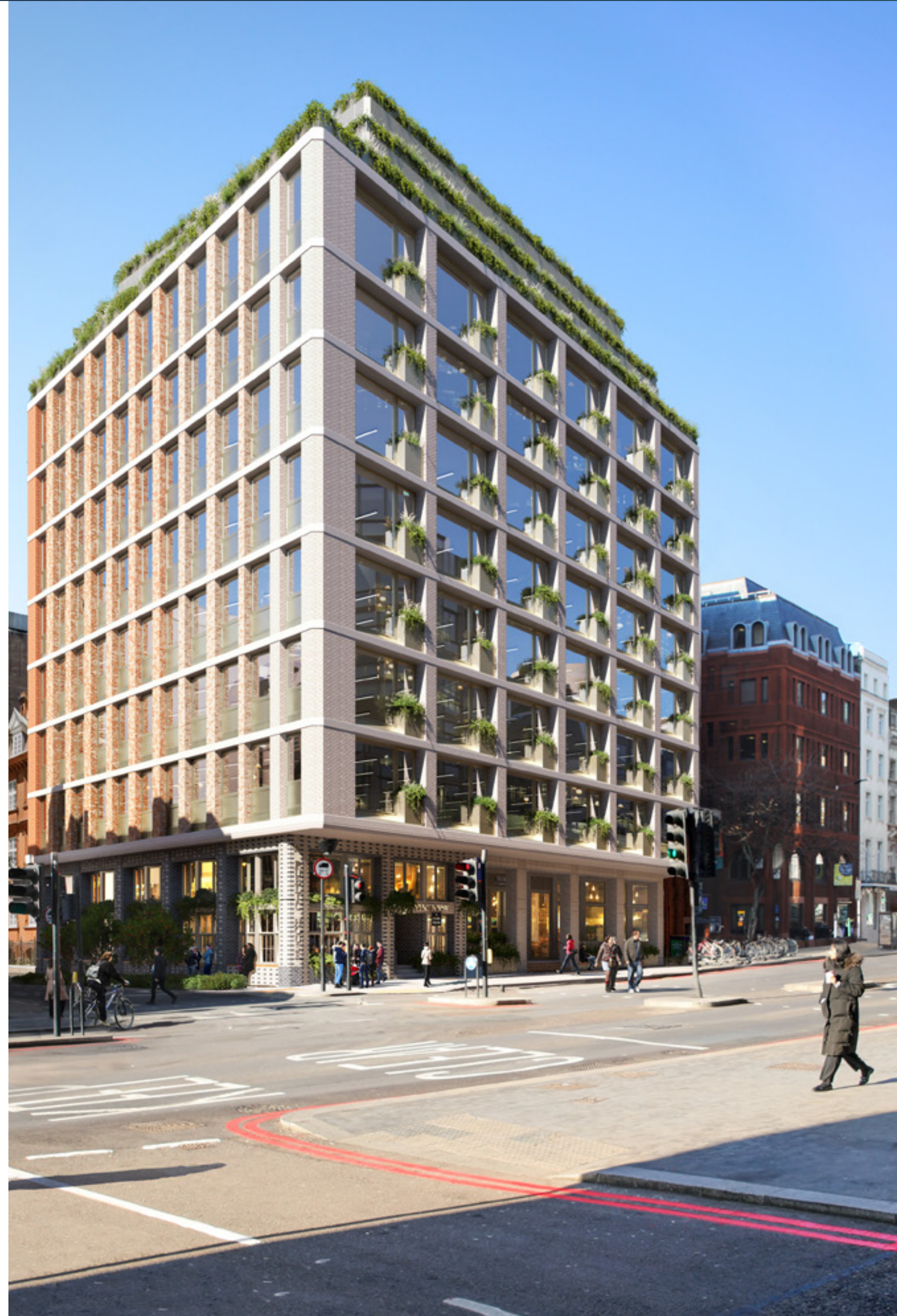
10 New Bridge Street, Royaume-Uni
